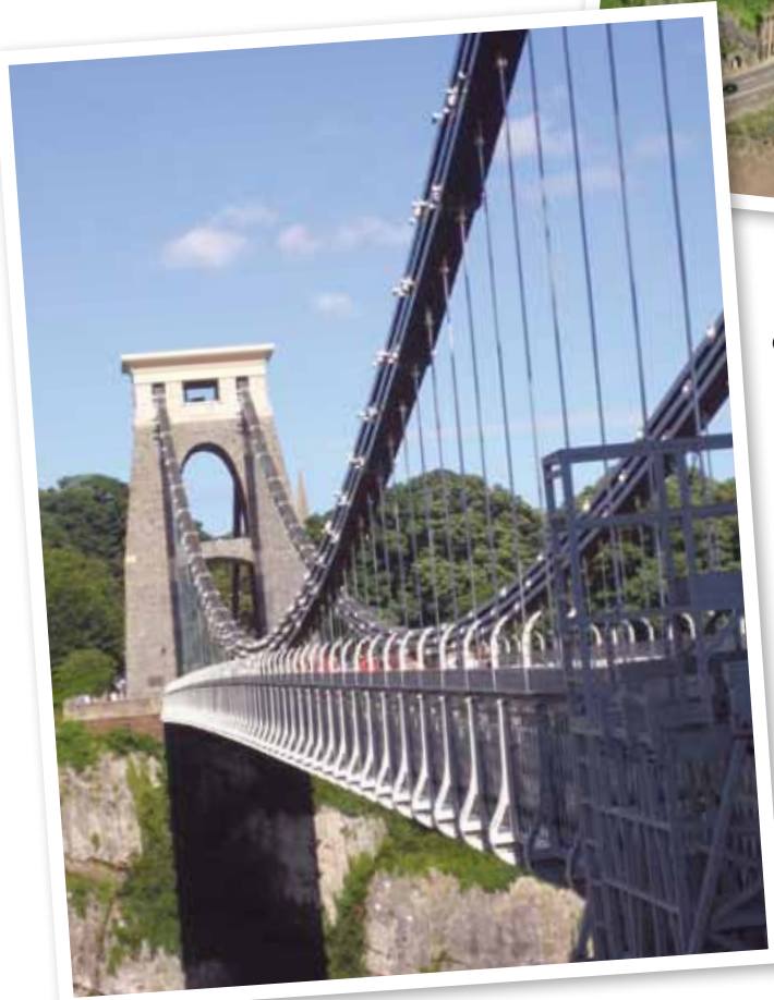
Most Clifton Suspension Bridge
